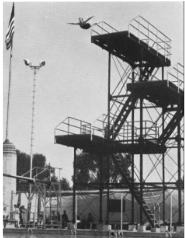
TEN METRE STEEL DIVING TOWER, SHOWING SAFETY STAIRWAYS
