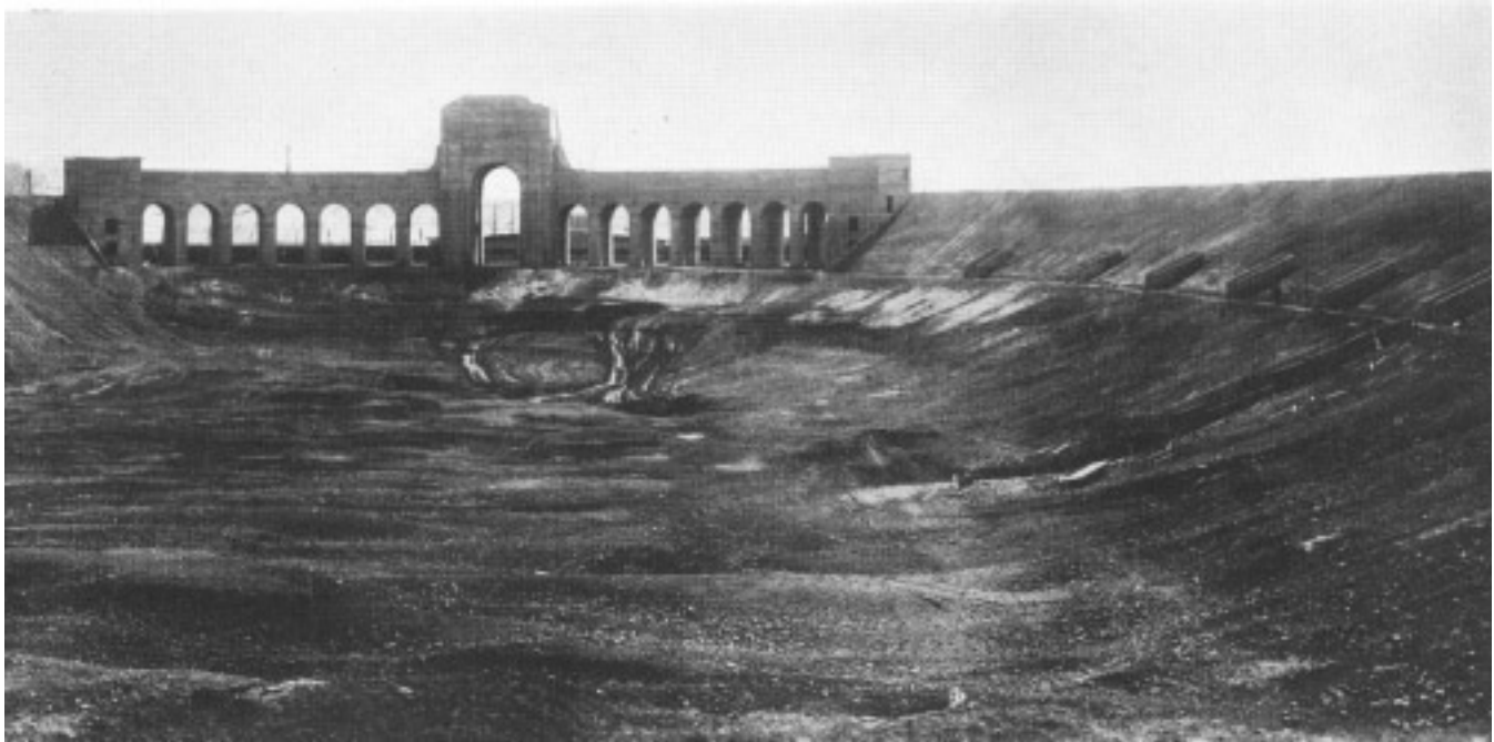
PERISTYLE AND EXCAVATION FOR STADIUM BOWL, 1922
