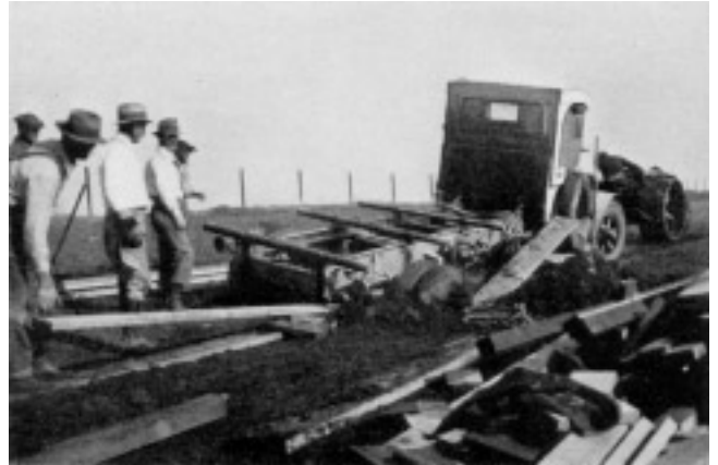
HEAVY RAINS IMPEDED THE WORK
