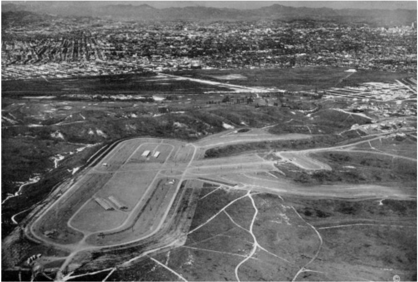
THE GROUND PLAN COMPLETED
