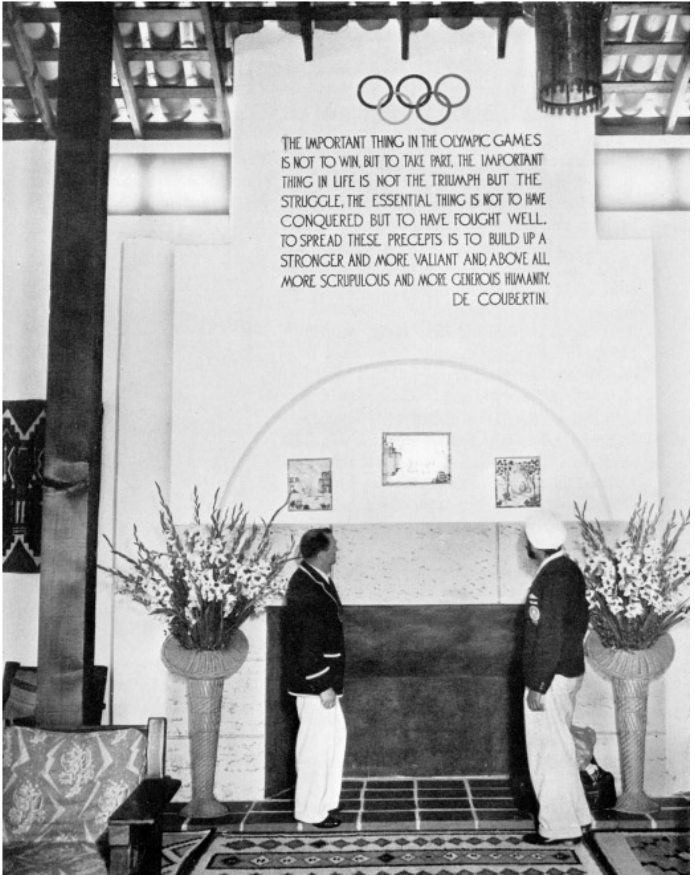
IN THE LOUNGE, ADMINISTRATION BUILDING, THE HEARTHSTONE OF THE VILLAGE
