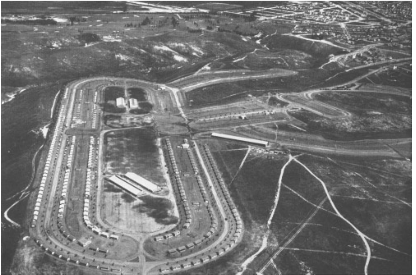
FIFTY HOUSES A DAY BEING ERECTED
