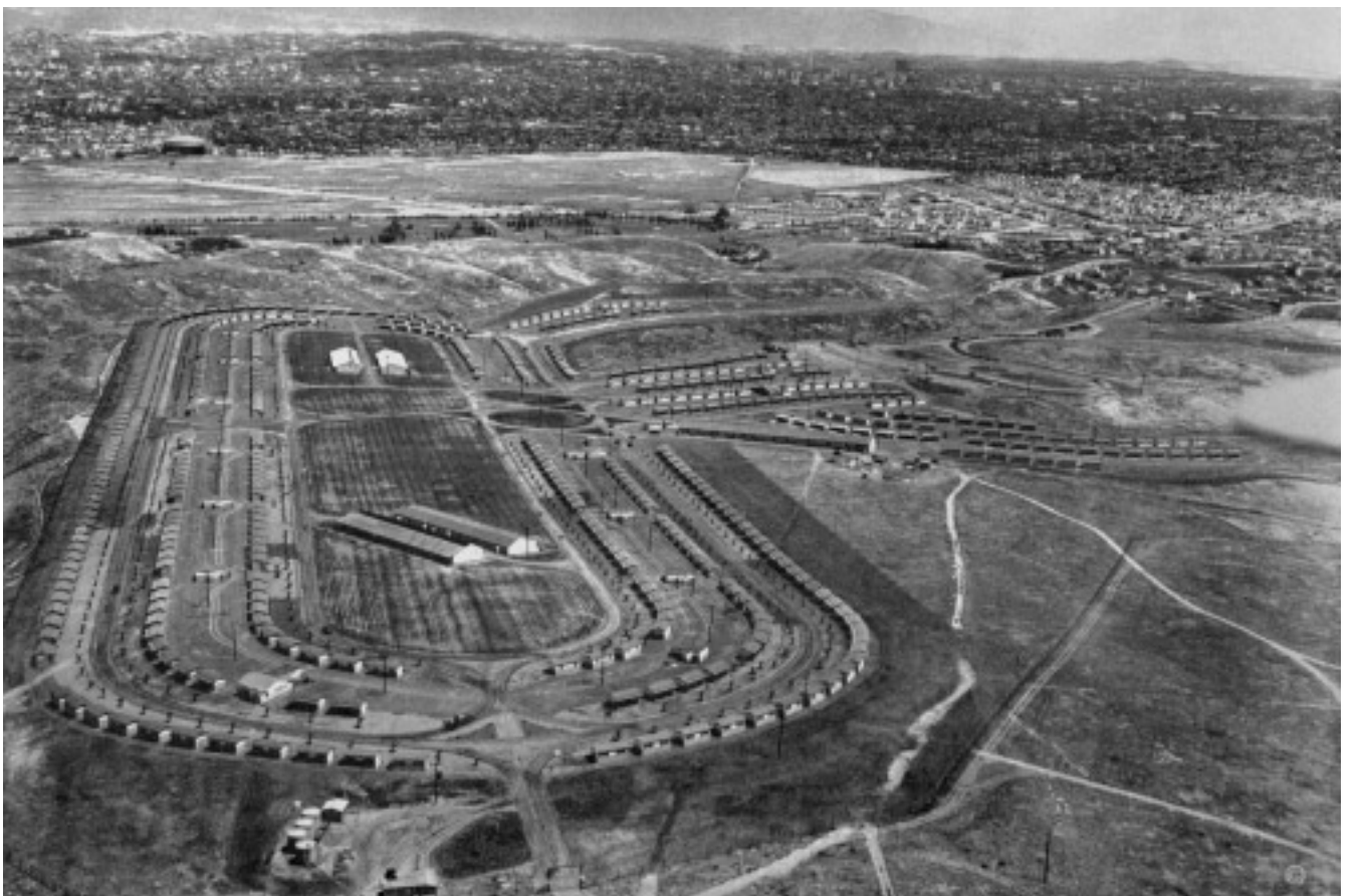
HOUSES AND DINING ROOMS COMPLETED
